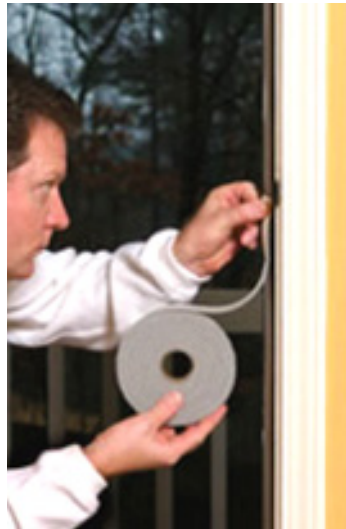
Applying Self-stick Foam Weatherstripping
