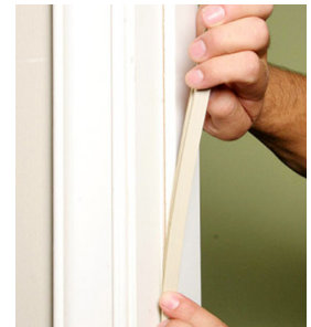
Installing Press-In Compression Insert Weatherstripping
